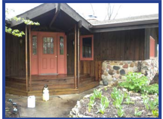
BEFORE AND DURING STRIPPING
