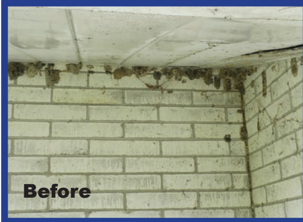
(above) Removal of mud nests in soffit corner
