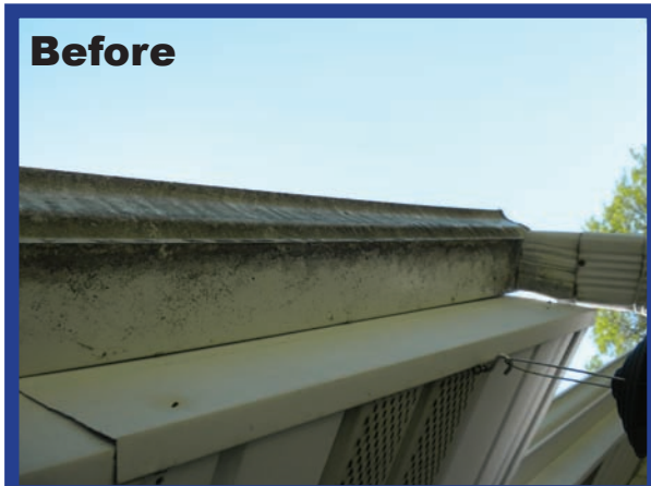
(above) Heaving mildew buildup and removal on gutters
