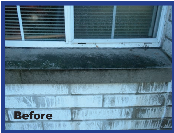
(above) Algae and mildew on window sill and removal
